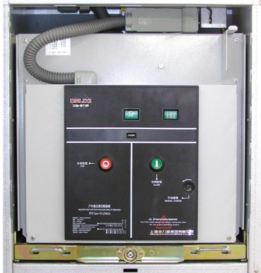
Figure 10. Movable component of circuit breaker in the testing/isolation position
