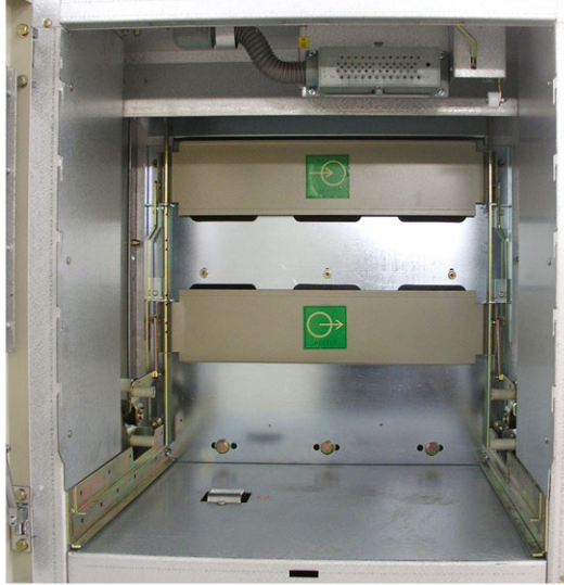
Figure 2. After the draw-out circuit breaker is moved, the static contact in the separate room will be shielded by the metal valve, the circuit breaker will be protected.
