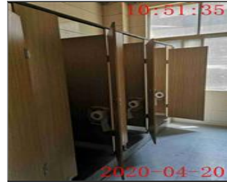
Photo of the sanitary facilities Washing room.jpg
