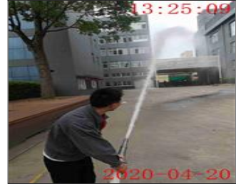
Photo of fire safety equipment Tested fire hydrant.jpg
