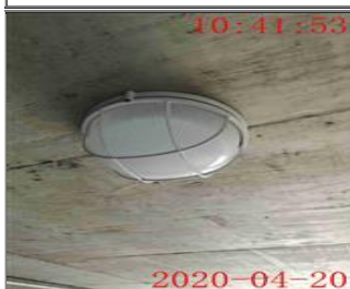
Photo of the inside of the main production hall Anti-explosive light installed in the chemical warehouse.jpg
