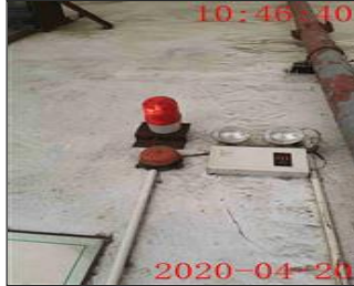
Photo of fire safety equipment Tested fire alarm.jpg
