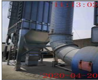
Photo of the inside of the main production hall Air emission treatment equipment.jpg
