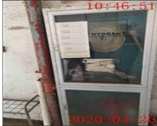
Photo of fire safety equipment Fire hydrant and fire extinguishers 2.jpg
