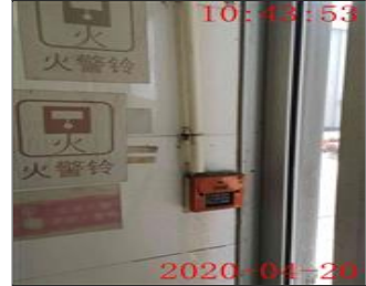
Photo of fire safety equipment Fire alarm.jpg
