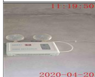
Photo of the inside of the main production hall Emergency light installed in the staircase.jpg
