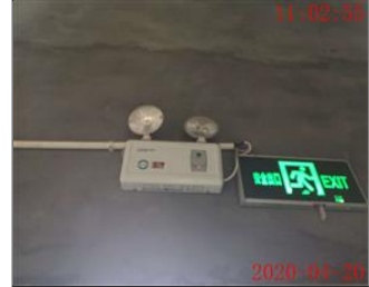
Photo of fire safety equipment Emergency light and exit sign 2.jpg
